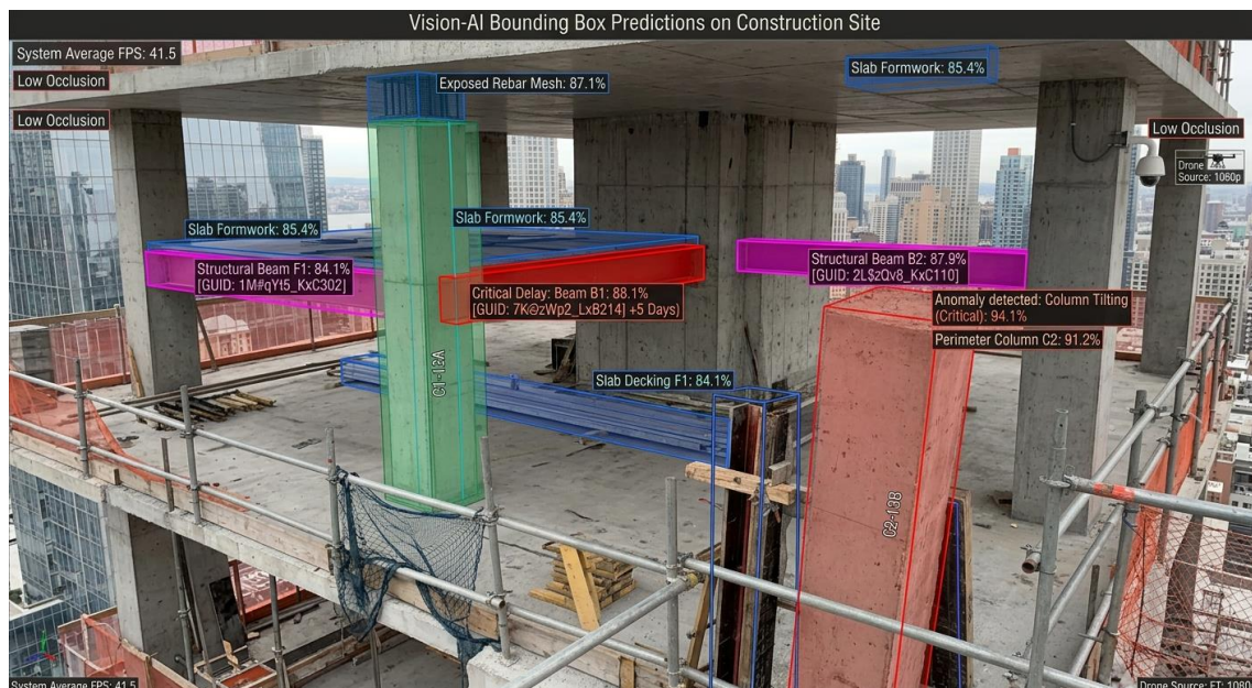
Figure 3. Vision-AI Bounding Box Predictions on Construction Site Visuals
